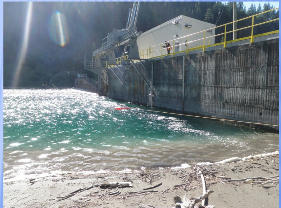
Hydraulic Measurements at Aberfeldie– Guideline Deployment
